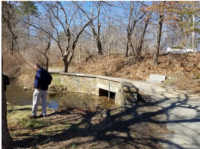
*Build up of debris in the culvert at the north end of Sargent Pond has led to failure of the culvert headwall.*
