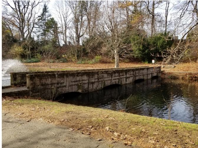
*Build up of debris under the Dickson Bridge deck has resulted in spalling, cracking and delamination of the concrete.*
