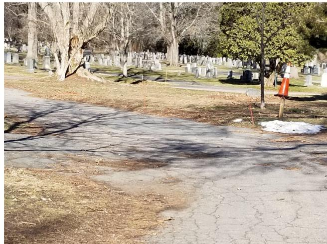
*Bituminous pavement throughout the cemetery shows signs of water build up resulting and cracks and failure.*
